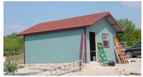
Gabriella's house nearing completion — Jimenez, Coahuila, Mexico, September, 2005
