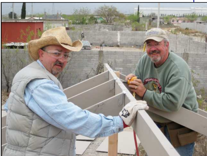
I wanted to prove that I actually did a bit of work in March! This photo shows Raymond Davenport of Quitman, Arkansas, and me as we nailed roof rafters in place on the Monclova house.
